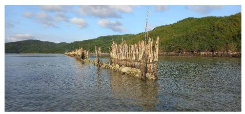
Figure 9. Stone reinforcement in the wave attenuation fence in Site 3 in Bagongon
