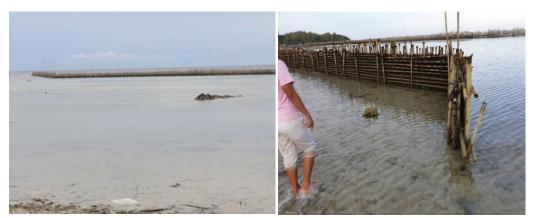
Figure 7. Wave attenuation fence (left) and sediment trapping fence (right).
