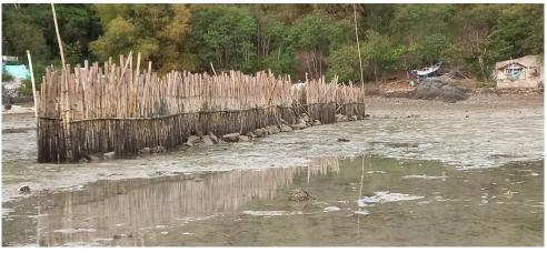
Figure 8. Stone reinforcement in the wave attenuation fence in Site 1 in Bagongon
