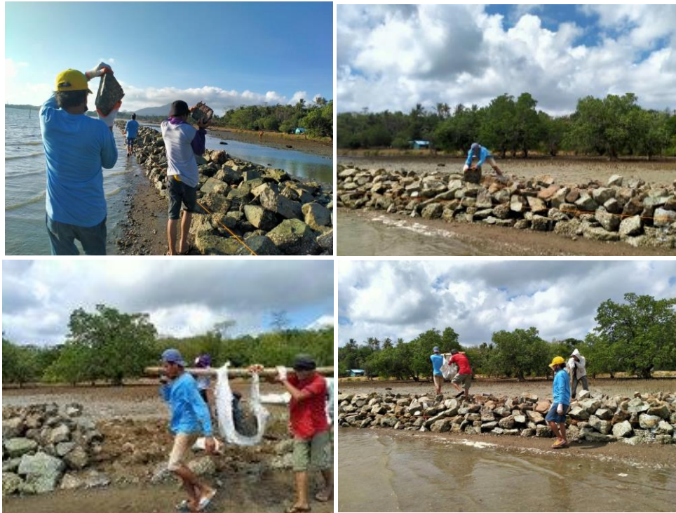
Figure 4. Manual piling of stones by TFO members during low tide.
